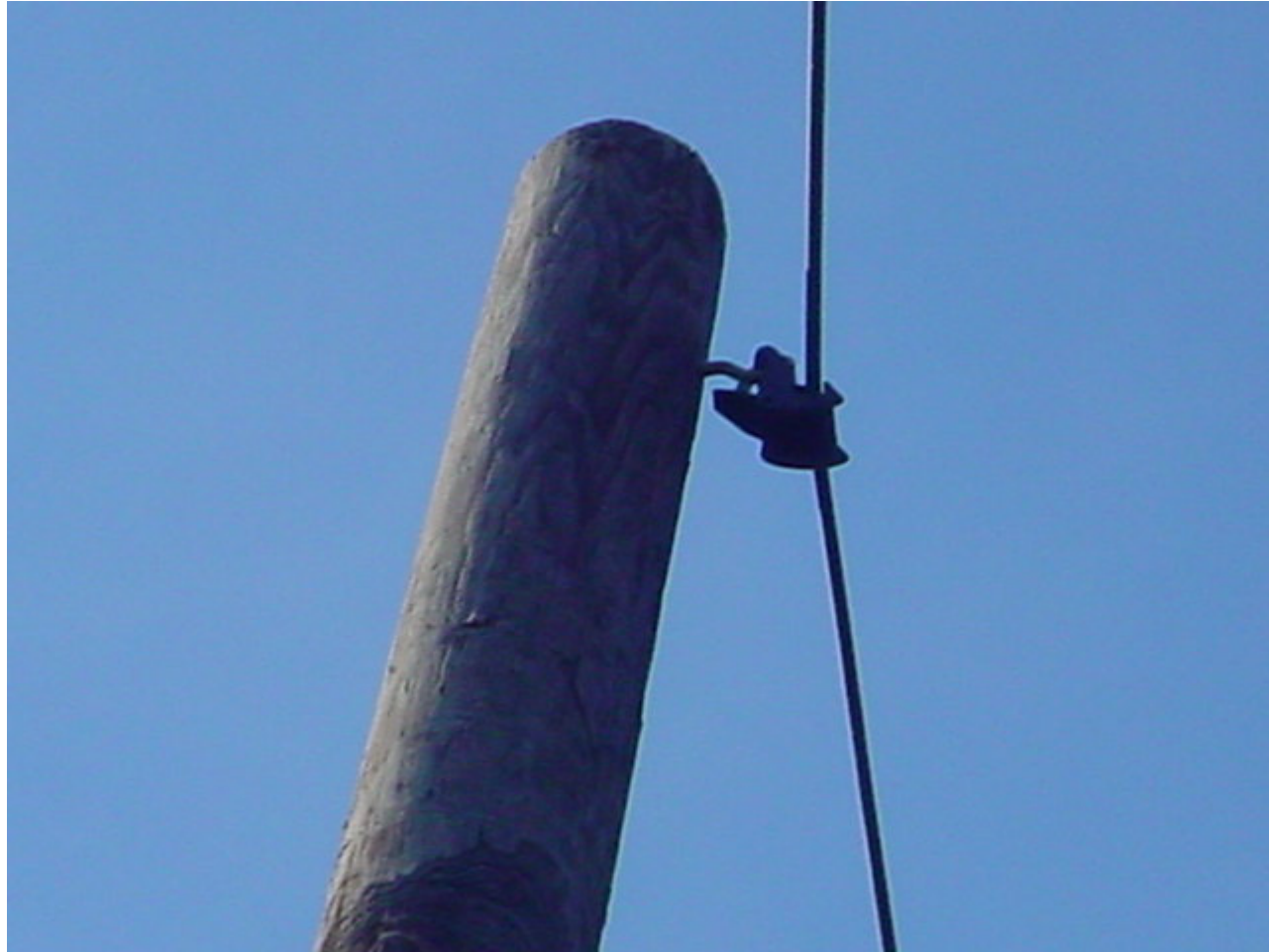
Concentric intermediate clamp.
