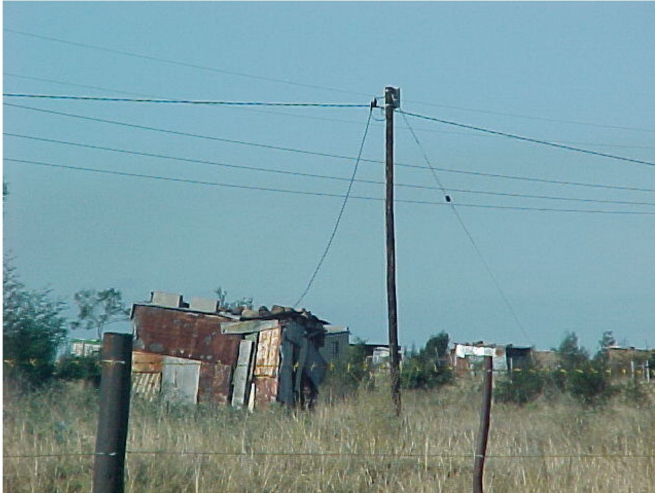
LV ABC with concentric service from a 2 way service box.
