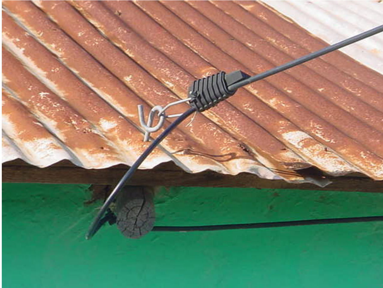
Concentric termination - wedge clamp
